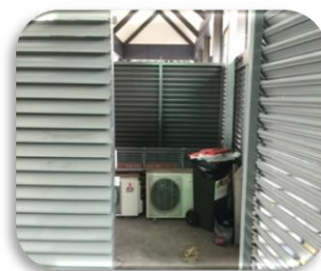
Inside the Lift Room
