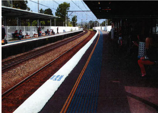
Photo 2: Typical curvature of station platforms.
